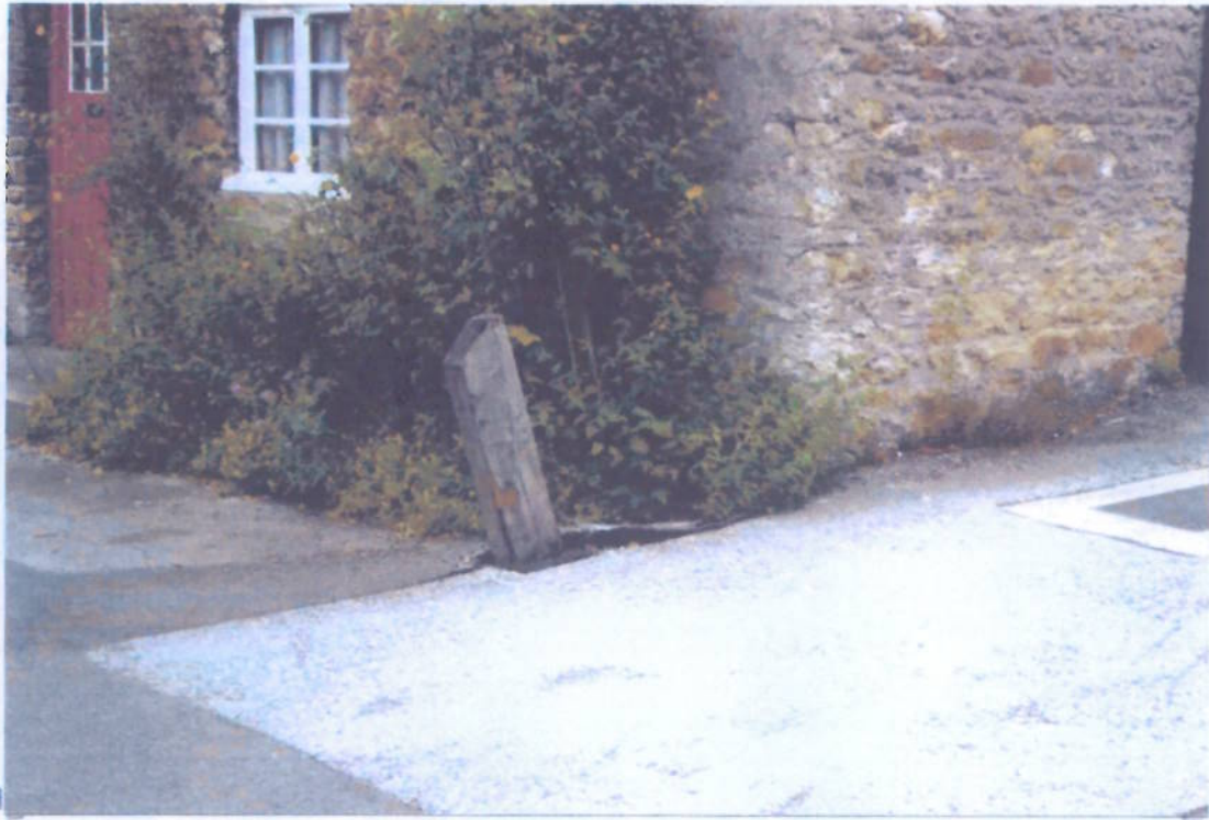
FIGURE 3: WOODEN POST AT CORNER OF N o . 53 POSITIONED TO PROTECT COTTAGE.
